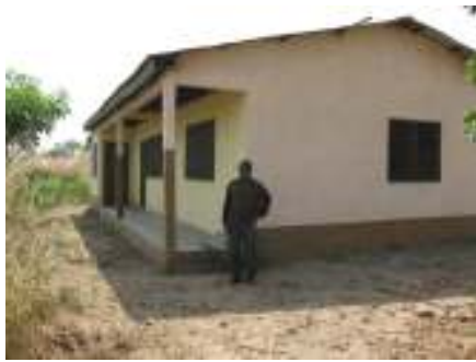
completed Kabeso clinic
